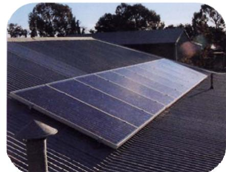
As detailed in the Photovoltaic Array - Calculation Methodology, there is a 3.6 year payback with a \$10,500 implementation cost and \$2,900 annual savings.
